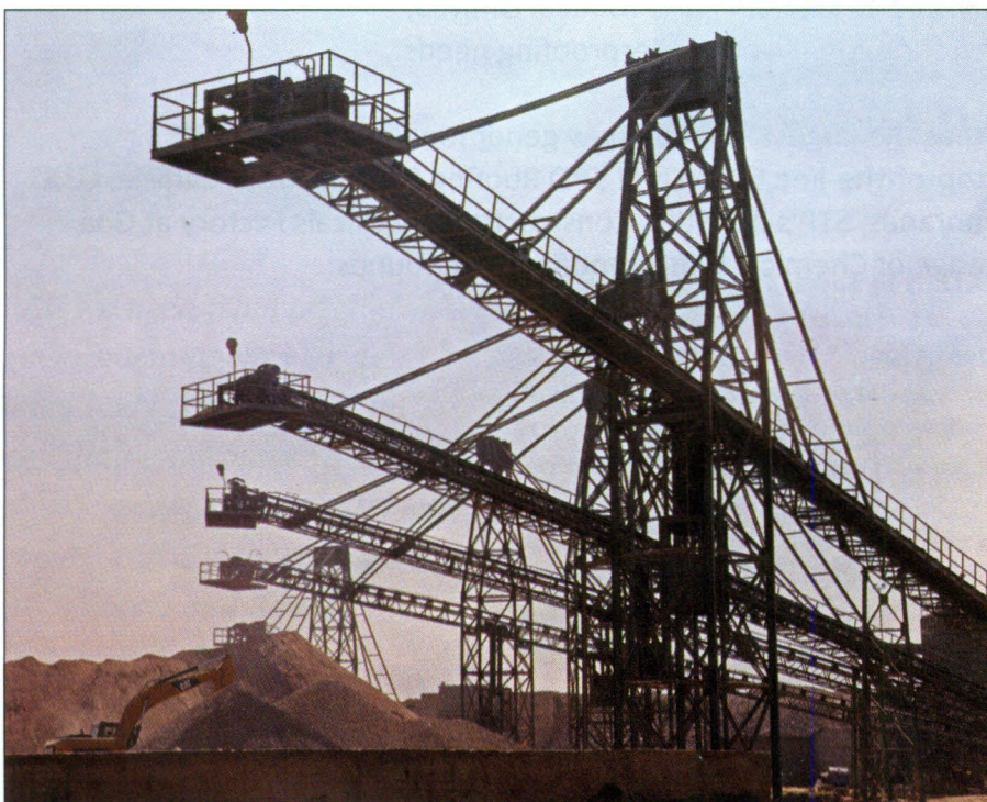
Work in full swing at Yamuna Expressway
